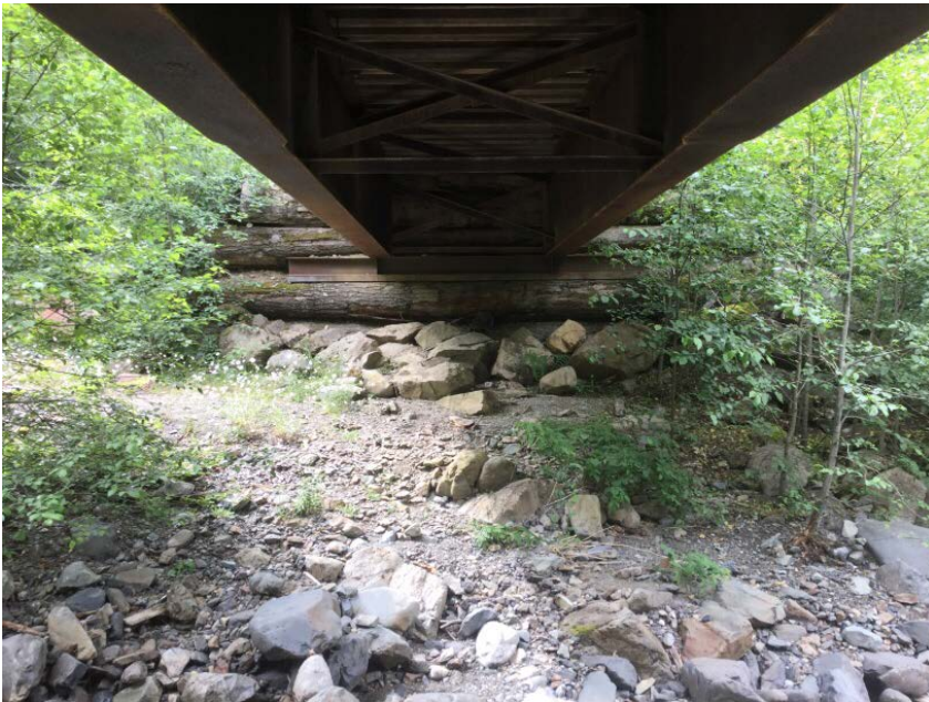
Left Bank Abutment when facing downstream
