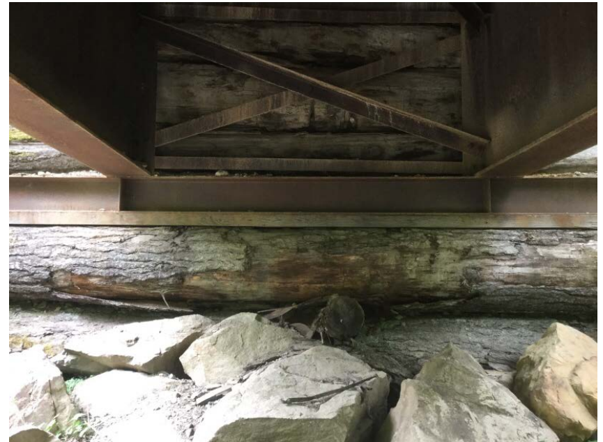
Left Bank Abutment when facing downstream
