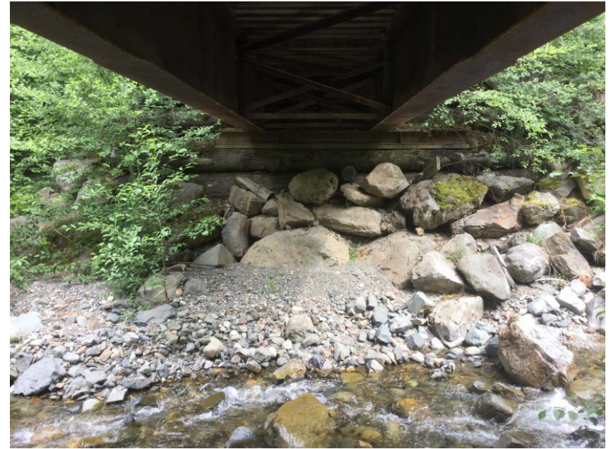
Right Bank Abutment when facing downstream
