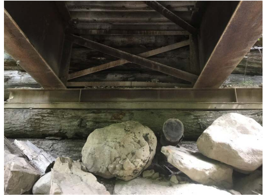
Right Bank Abutment when facing downstream
