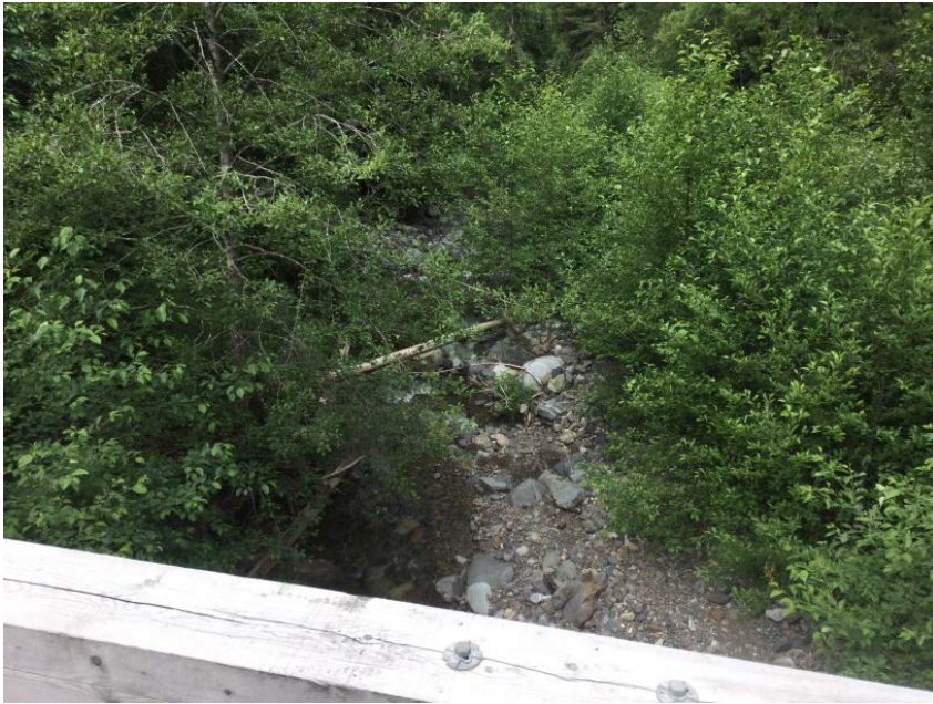
Looking downstream from deck
